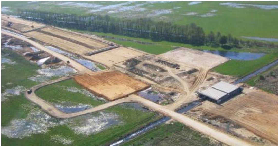
Figure 5. Aerial view of the dynamic replacement platform at the bridge approach.
