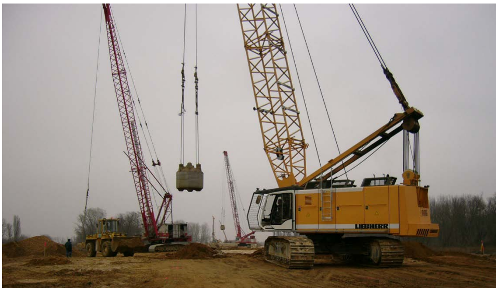
Figure 4. Application of dynamic replacement in the project.
