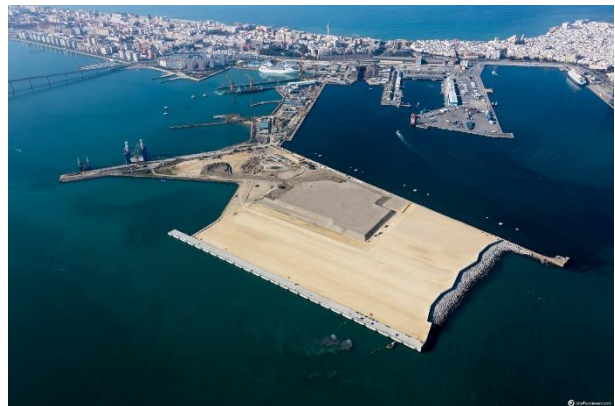
Figure 1. Cadiz port. During the third phase preload.
