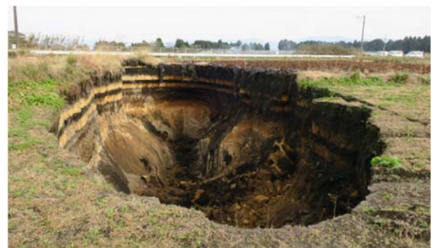
Figure 1. View of the sinkhole
