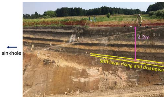
Figure 10. A stiff layer in the west of the sinkhole
