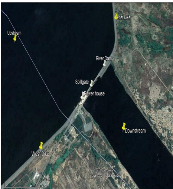
Figure 1: The Kpong hydroelectric dam (Source: Google earth)
