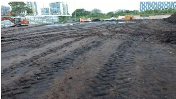
Figure 3. Embankment after completion.
