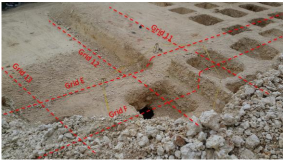
Figure 8. View of the footing excavations with grid lines (Survey 2)
