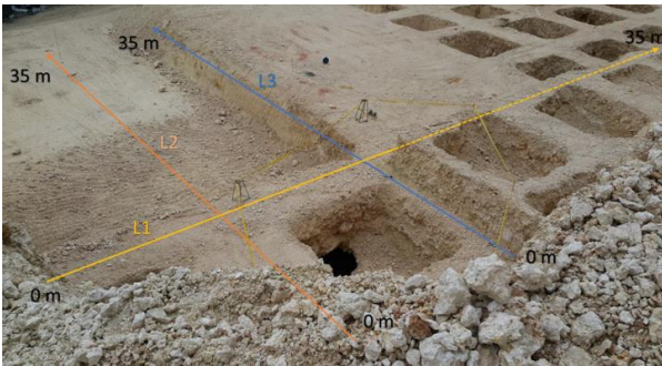
Figure 10. View of the footing excavations with grid lines (Survey 3)
