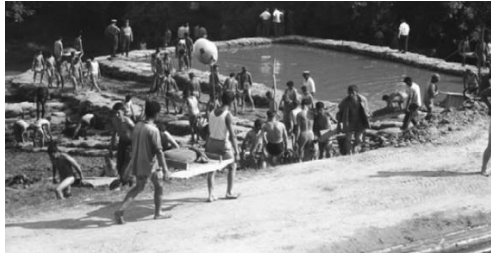
Figure 10. Danube, Margitta Island piping, counter-pressure and diaphragm walls at the waterside, the cause was the vicinity of an old meander, Horváth 2001
