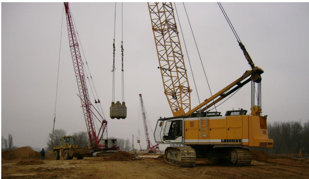
Figure 4. Application of dynamic replacement in the project.
