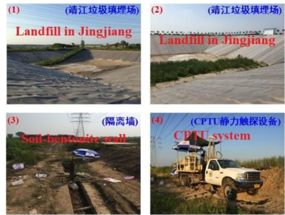
Figure 2 Landfill and soil-bentonite wall
