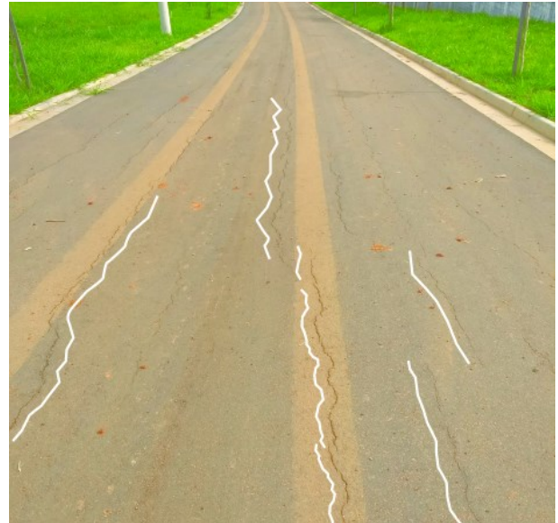
Figure 4. Typical Longitudinal crack in the site study.
